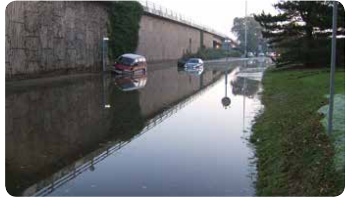
200mm PVC water main burst.
