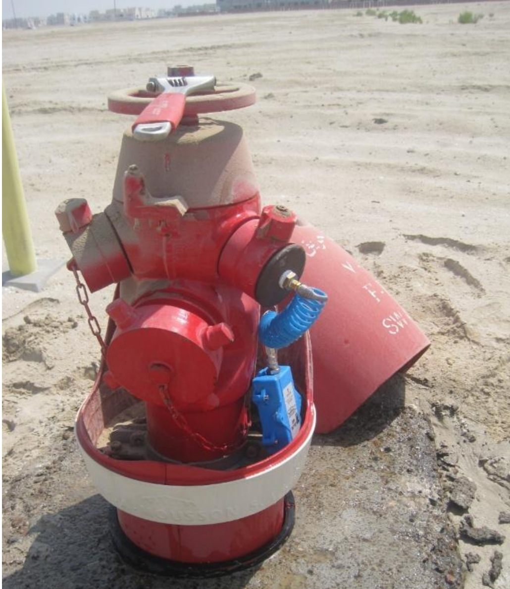
Temporary Pressure Logging inside a DMA in UAE
