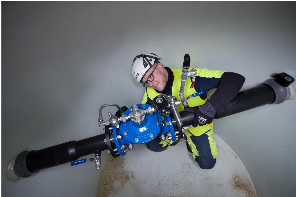
Installing Brand New DMA Inlet Chamber with PRV
